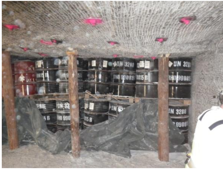
Fig. 6: Photo of waste drums in emplacement gallery; the degradation of the roof started to bear down on them [13]
